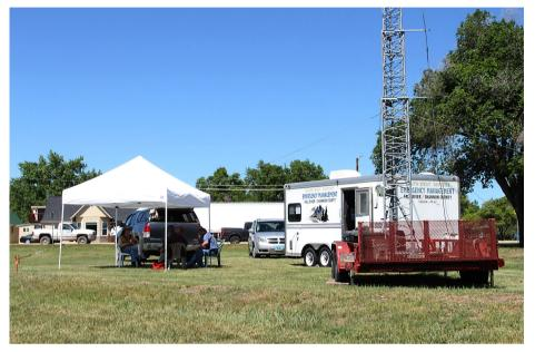
We secured the tower trailer to the ground with steel cables and attached them to steel stakes that we pounded into the ground! After that we unloaded the antenna, assembled it and attached to the tower on the trailer.
